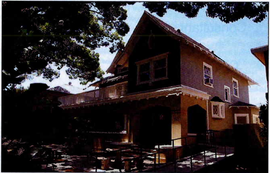
Isaiah House in Santa Ana was kept open due to the joint efforts of several legal firms and updated by volunteer contractors
